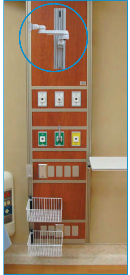
Monitor Channel mounted on vertical headwall - SSM Monitor Arm mounted on channel
